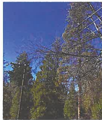
Inspection photos show tree branches that came into contact with wires featuring the protective coating (covered conductor). Power remained safely on for customers in the Idyllwild area of Riverside County - Nov. 25, 2021. Credit: Trenton Koury
